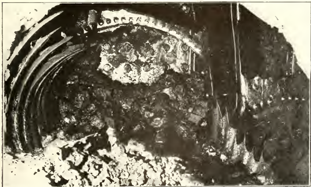
INJURY TO THE BOILERS OF SOME OF THE GERMAN LINERS REPAIRED BY R. D. GATEWOOD, '06, AT PANAMA THE DAMAGE WAS CAUSED BY DRY FIRING
